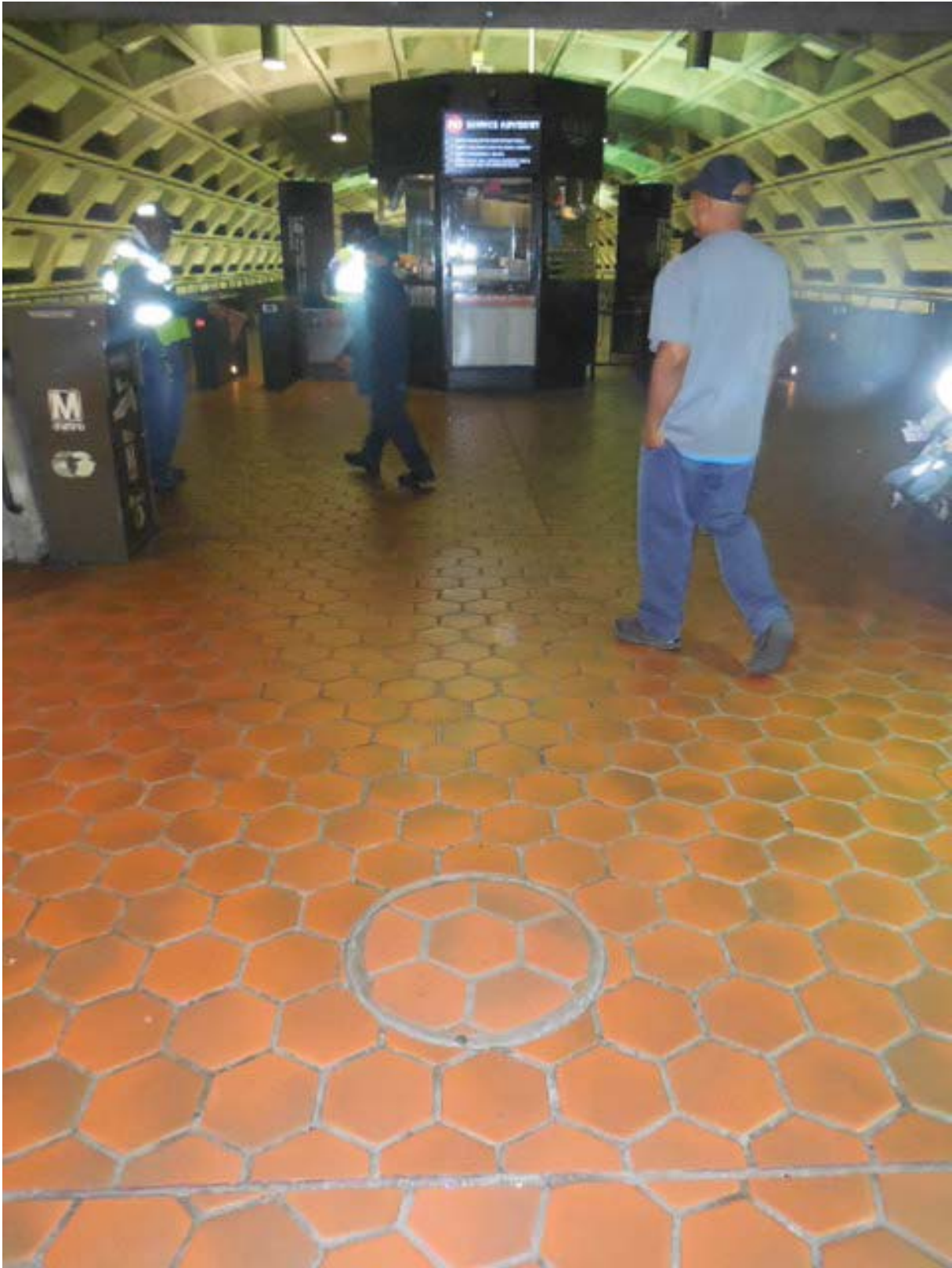
Picture 1: E03 U Street West – Intermediate manhole in mezzanine
