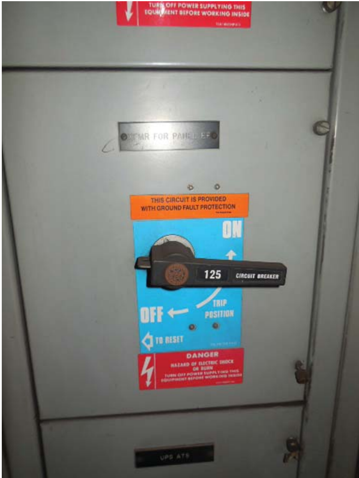
Picture 9: E03 U Street East – Essential SWBD Transformer in Room 109
