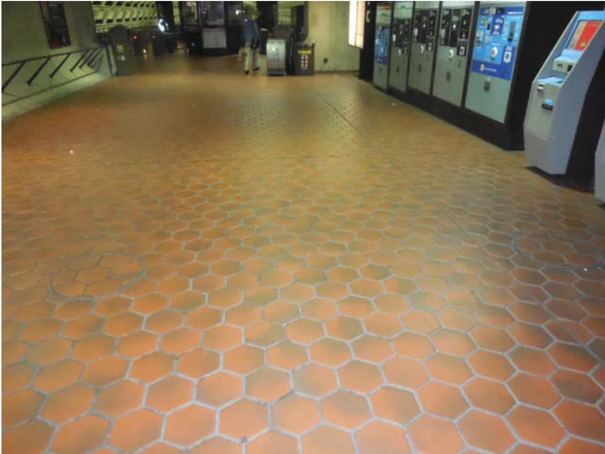
Picture 2: E03 U Street East – Mezzanine manhole
