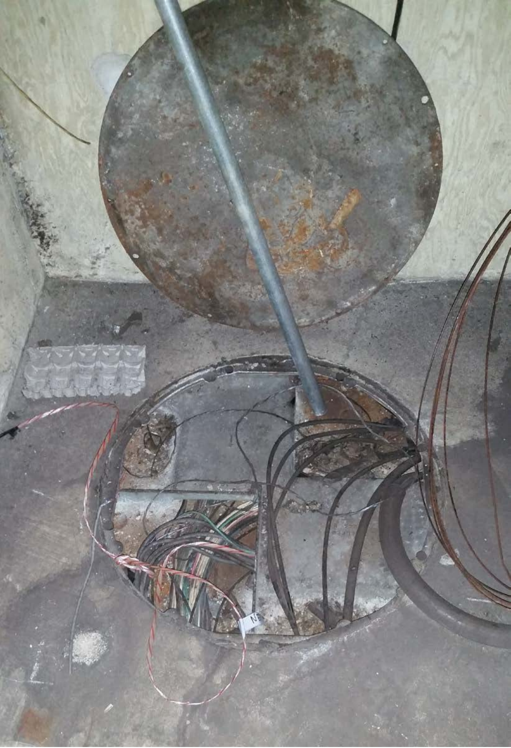
Picture 2: E05 Georgia Ave – Manhole in room C213
