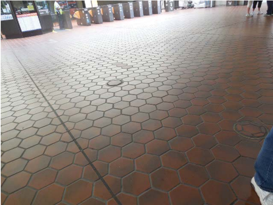
Photo #2: E10 Greenbelt – Handholes at Mezzanine
