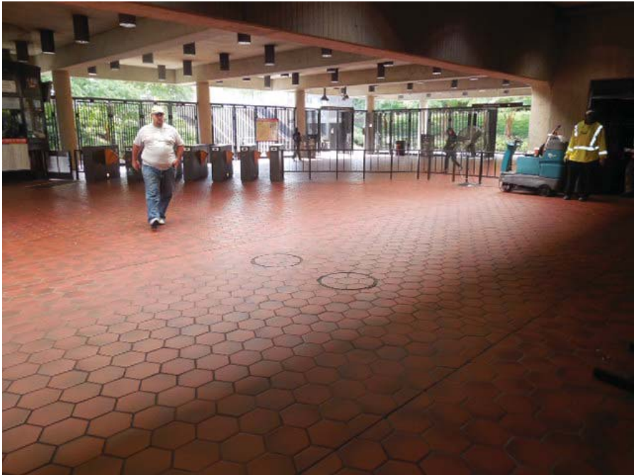
Photo #1: E09 College Park – Handholes in Mezzanine Floor
