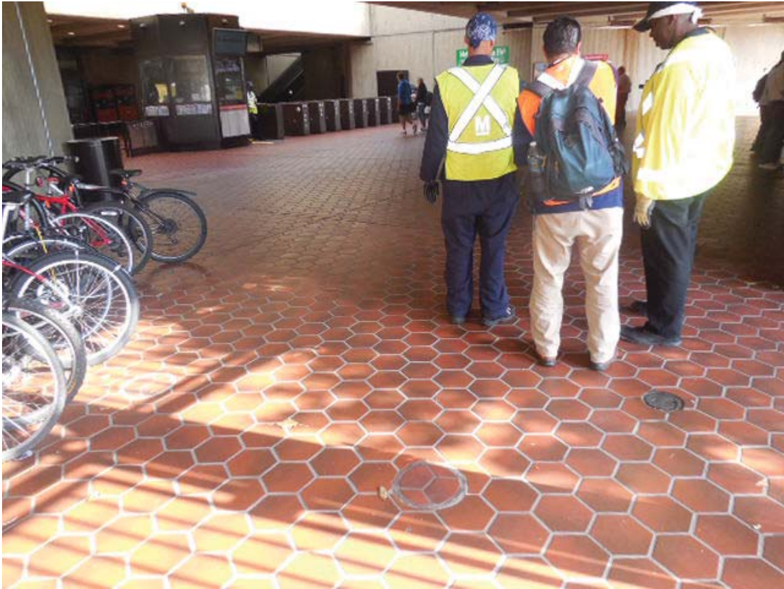
Photo #1: E10 Greenbelt – Handholes at Mezzanine
